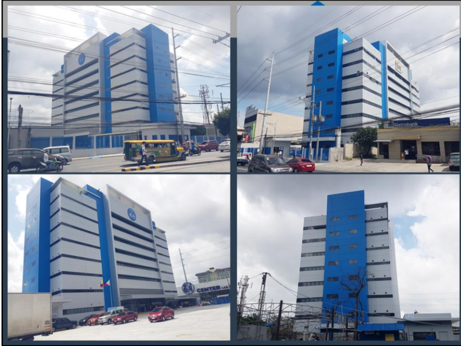
These are photos of the façade showing all four sides of the building.
